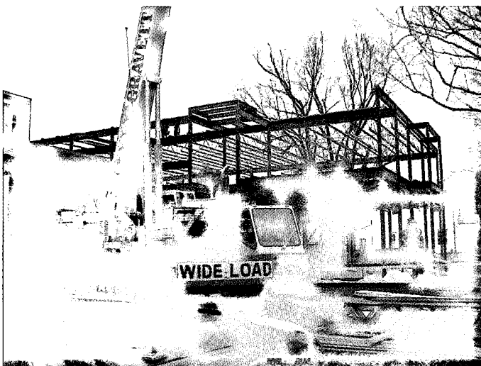
It's going up! The erection of steel for the new addition.
